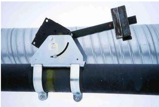
**Figure 8. Picture of the Installed TVA on the arctic pipeline (above pipeline configuration).**
