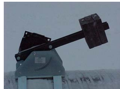
Figure 3: Top-of-Pipe Tuned Vibration Absorber (TVA) Device
