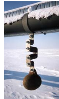
Figure 2: Typical Pipeline Vibration Damper (PVD) Device
